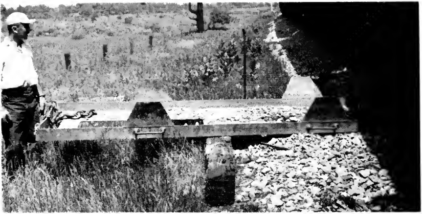
Ballast unloading pan.
